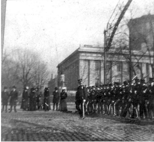
The Hibernian Rifles march up High Street in front of the Statehouse.
